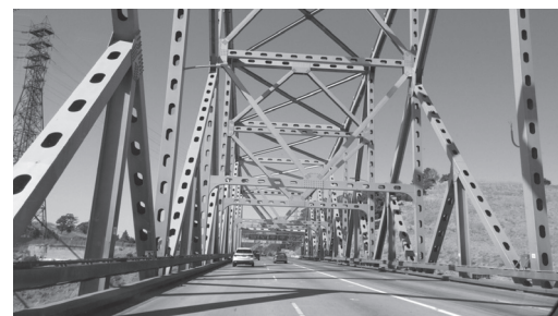
Struts with perforated cover plates used in the Carquinez cantilever truss bridge (East bound I-80), California, USA
