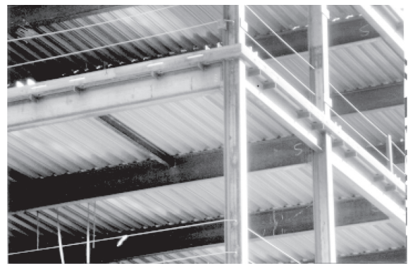
Close-up view of the column of the above building (Note the composite slab)
